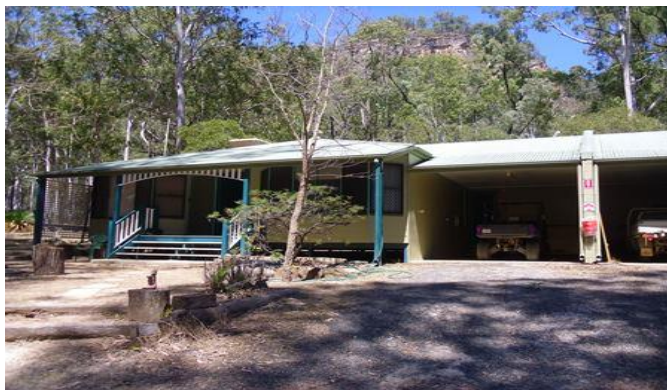
(Front view of eastern duplex)
